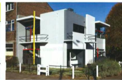
Figure 2.2.8 'Schroeder house' by Gerrit Rietveld, 1924.
